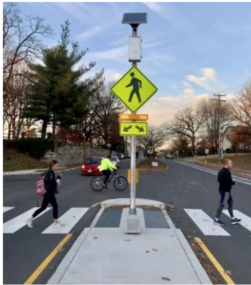
Pedestrian Refuge Island with Beacon
